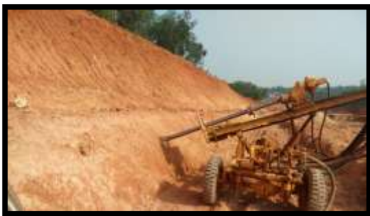
1.1. Drilling of Soil Slope
