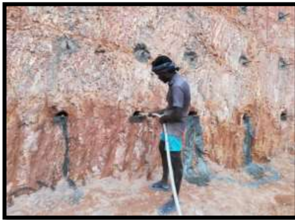
1.3 Shotcreting with cement slurry
