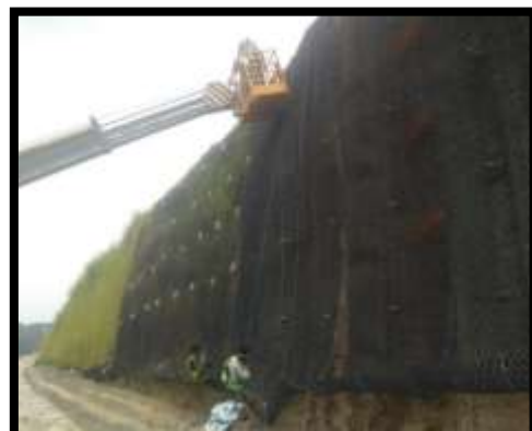
1.7. Installation of Geo-grid
