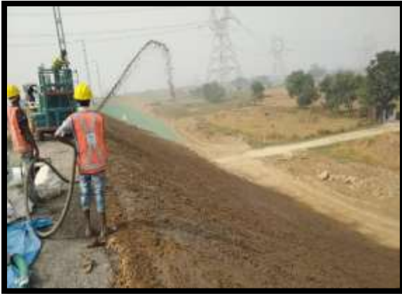
1.4. Spraying of seed slurry
