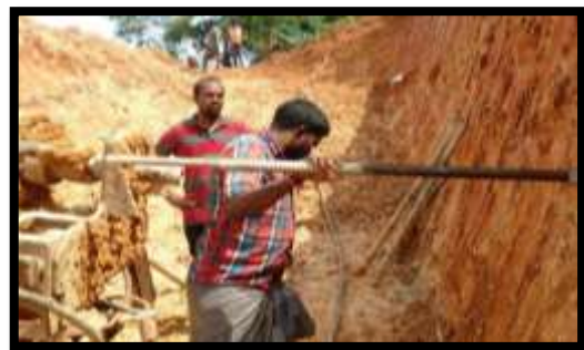
1.2. Insertion of Dowel bars into
