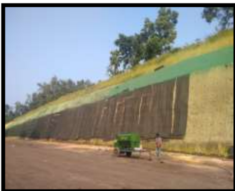
1.6. Geo-grid in hill slopes
